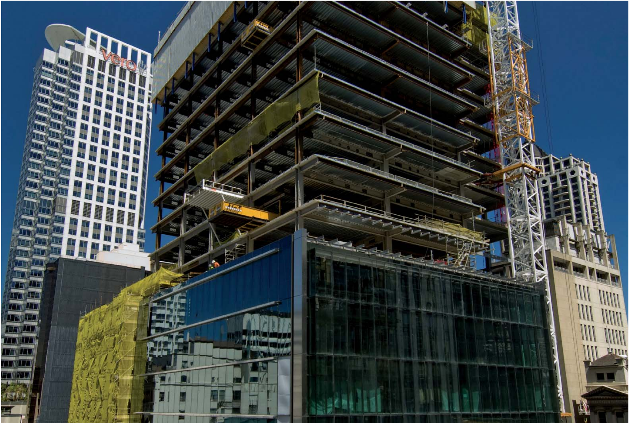
ComFlor 80 in construction at 80 Queen Street, December 2008
